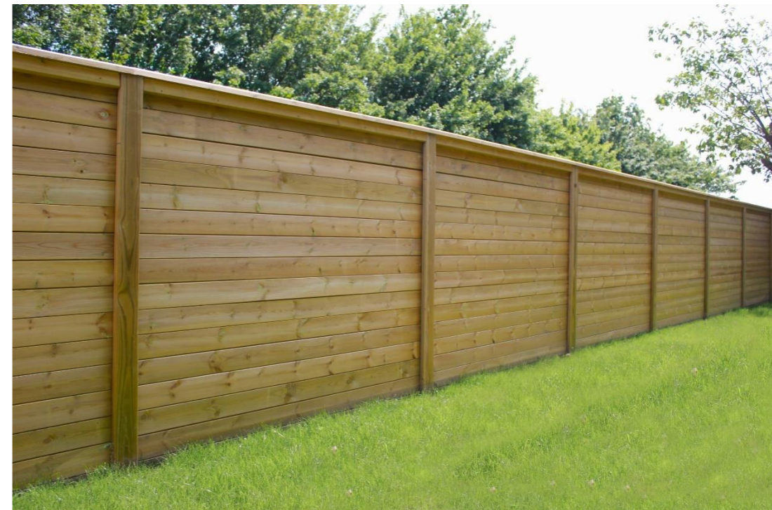
Fig 56. Illustrative example of the use of close boarded acoustic timber fencing
